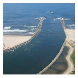
tidal currents in the inlet, allow very little sand to flow across the inlet. Material that does pass through or around the jetties contributes to shoaling either in the interior of the inlet or offshore, depending upon the direction of tidal flow.
