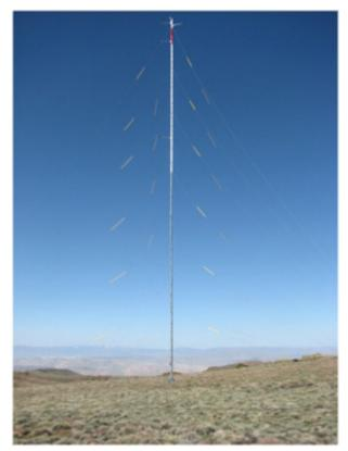
**Figure 5.** Typical 60-meter met tower found in Wyoming, which includes guy wire reflectors and a painted top for aviation visibility.
