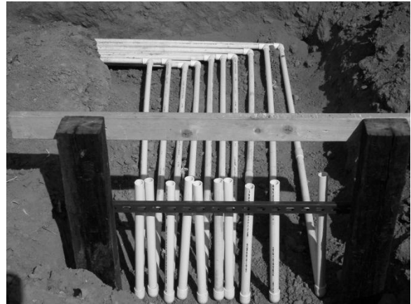
Figure 3. Installation of surface drip irrigation at PREC.
