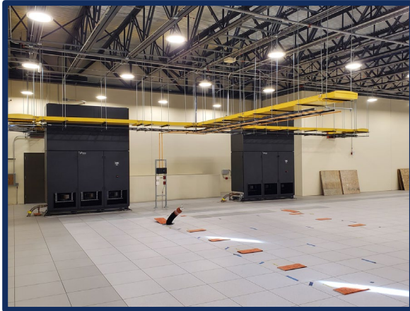
CRAC Installation for Derecho Air Cooled Load and CDU Hose Mock-up
