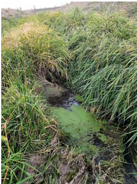
Figure 4. Overgrown vegetation on the ditch bank has slowed the water enough for duckweed to start growing.
