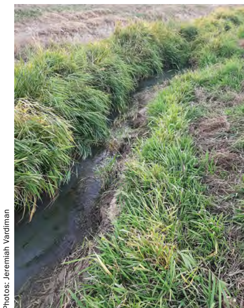
Figure 1. Sediment building up on the right side pushes the water channel to the left side.
